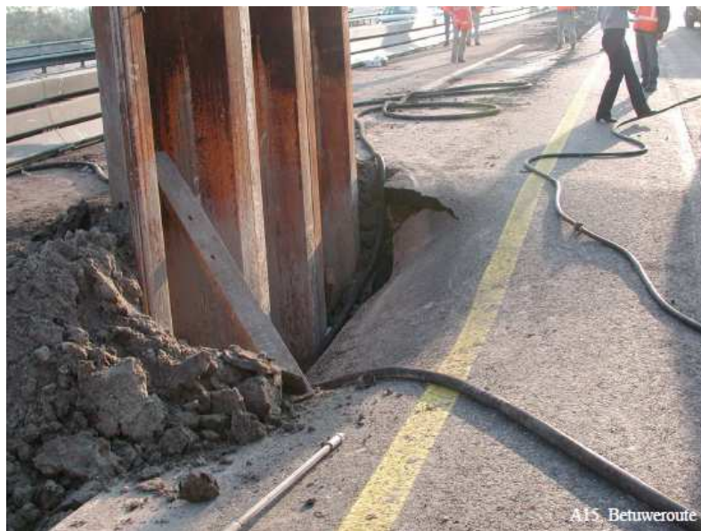
Figure 7.6: Example of the effects of vibrating sheet piling
